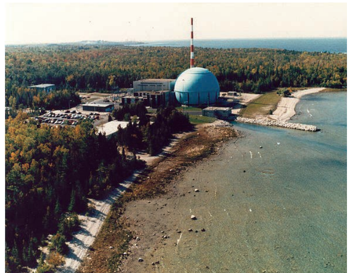
Fig. 20 Big Rock Point nuclear power plant in the US. Safety containment in the form of a large steel sphere was typical for early constructions.
