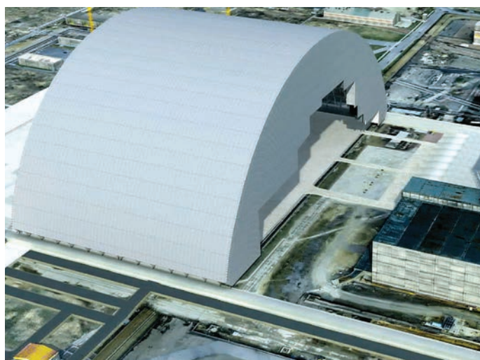
Fig. 34 Sarcophagus constructed by the NOVARKA French company (state as of April 26, 2014; source: http://footings.wordpress.com/2011/04/20/cannibal/ ).
