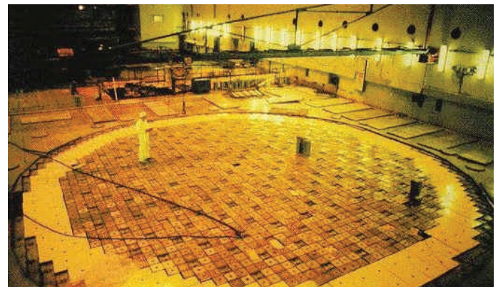
Fig. 33 RBMK reactor top view. Visible 25 x 25 cm squares hide 2,488 blocks of graphite moderator, 1,661 pressurized channels with fuel rods cooled down by flowing water, and 222 blocks with control rods.
