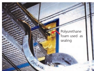
Fig. 30 Typical cable tray penetration (source: Wikipedia Commons).
